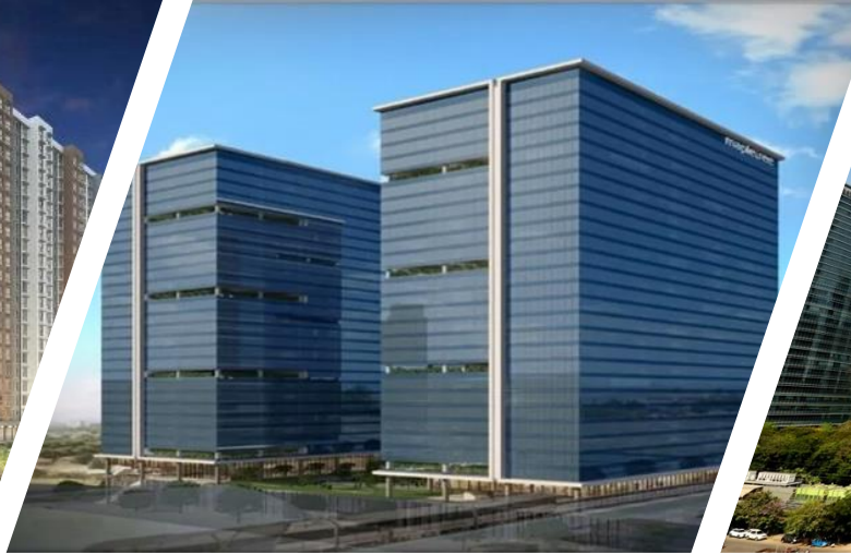
MAPLETREE THE FERN, VIKHROLI, MUMBAI L & W CONSTRUCTION PVT LTD Area: 29,40,043 Sq. Ft / 27 Floors
