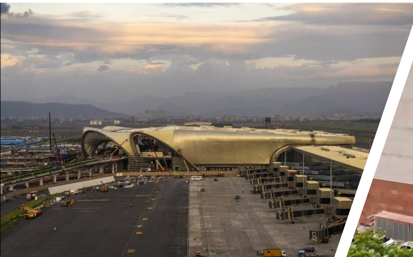
NAVI MUMBAI AIRPORT L&T CONSTRUCTION PVT LTD Area: 6,72,270 Sq. Ft. / G+2 Floors
